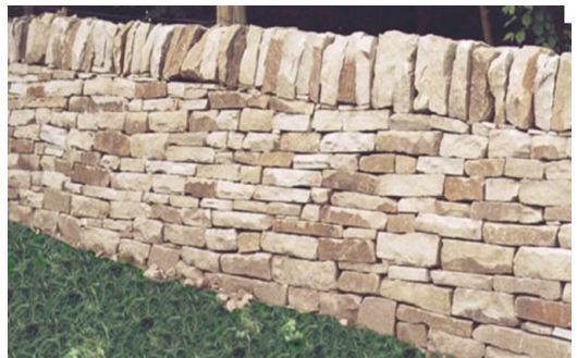
Sandstone—Cheshire coursed Dry Stone Wall
