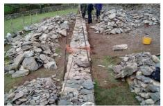
I then fill in between the stones with what we call **hearting**. I can then start to build the wall. This is called the first lift. I make sure that the stones are placed with the long edge into the wall. I have to build up both sides of the wall as I go and I make sure that each layer of stones is filled in with **hearting**.
