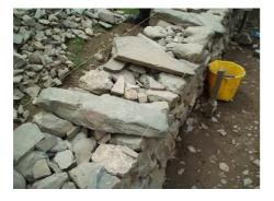
When the wall is about knee height, we put in **through stones**. As the name suggests these go right across the wall and sometimes stick out. They add weight to the wall and anchor both sides together. They can look like stepping stones but please do not climb over walls. Use gates or stiles. Climbing over walls can disturb and loosen the stones which makes them more likely to fall down.
